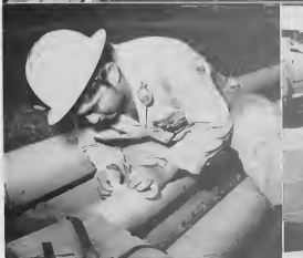
VICTOR THOMP, engineering assistant A, top left and above left, visually checks the inside of a gate valve and uses a depth gauge to measure wall thickness loss on a pipe. Employing an on-stream inspection technique, top right, is R. Gil who is testing corrosion agent in a product. At left and right are L. Giel and C. Polak, EIG inspectors, who are measuring shell and pipe thicknesses with Audigage, left, and Penetron, right.
